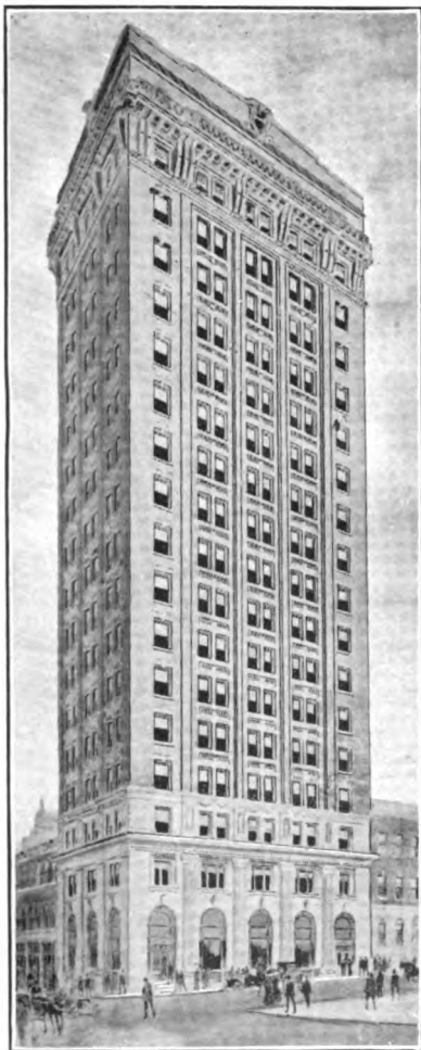
New Bank and Office Building which is to be opened soon by the Central Bank and Trust Company of Memphis, Tenn.
